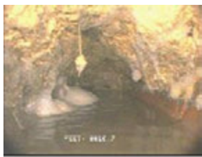
Grease on walls of a sewer pipe
