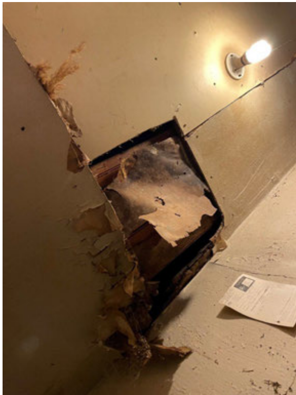
Photograph 6 – Attic entrance at 2708 Wayne St.
