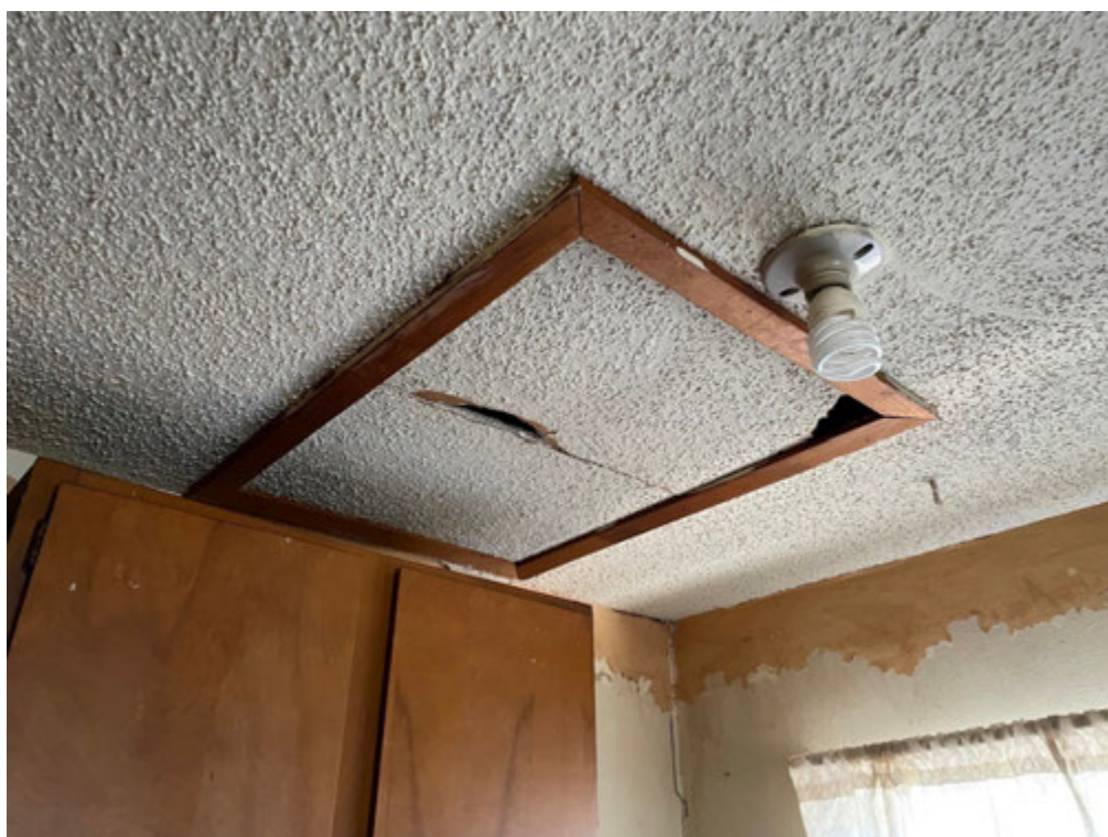
Photograph 2 – Attic entrance at 2811 Amboy St.
